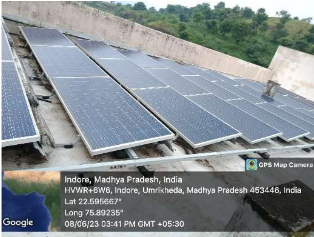
Fig.- 5.4 - 25 KWp PV Power Tech Solar Panels Installation
