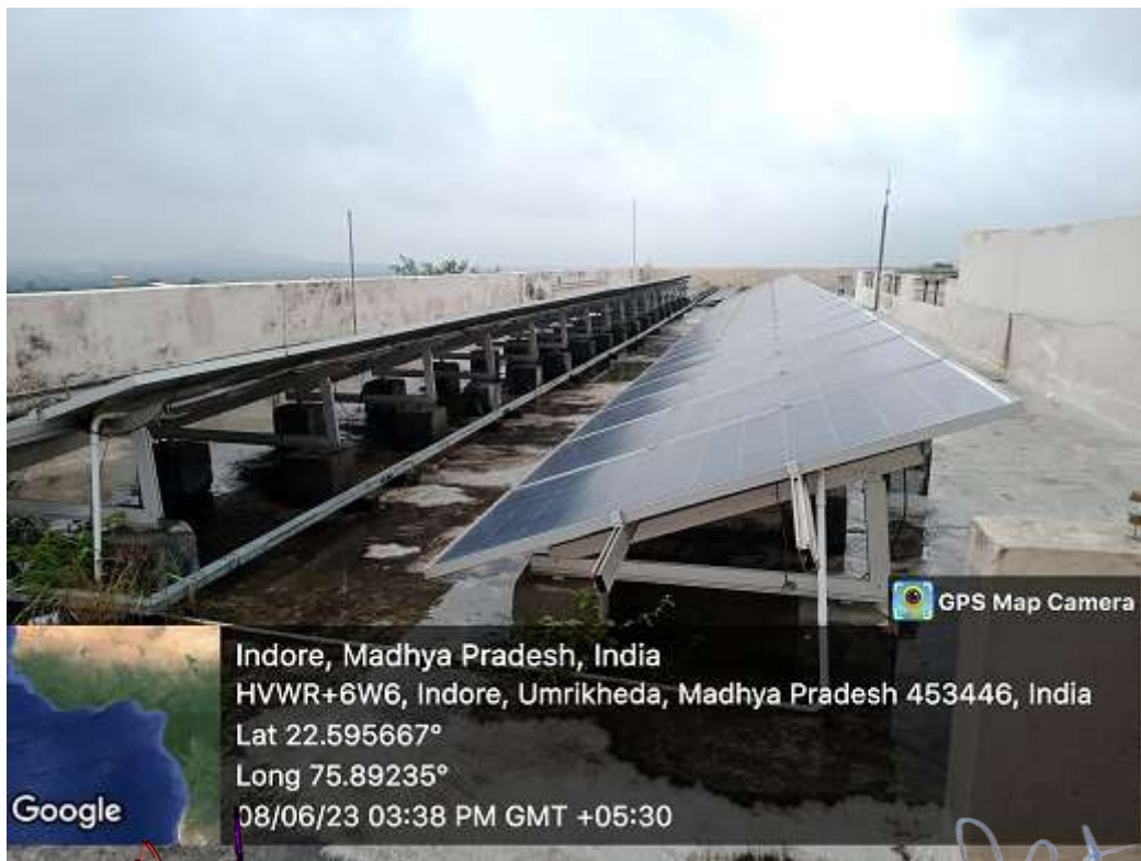
Fig.-5.5 25 KWp PV Renewsys Solar Panels Installation
