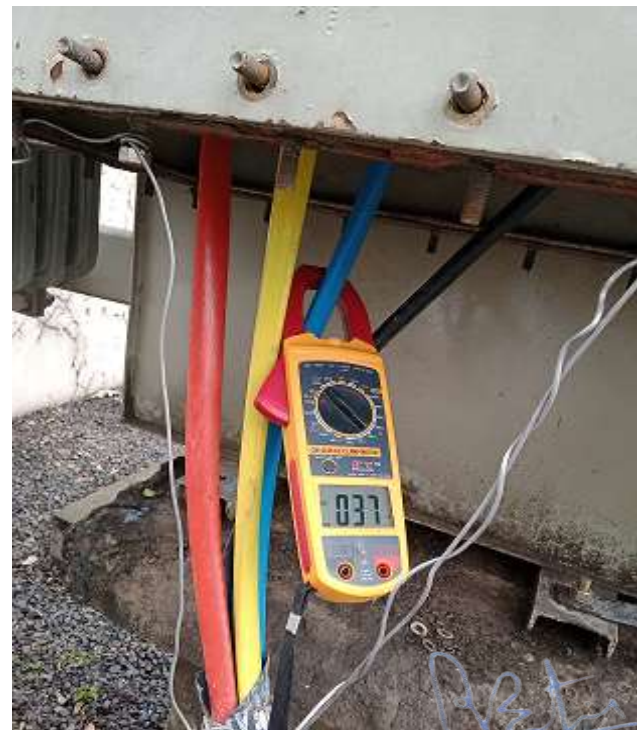
IQAC COORDINATOR Fig. 5.2 Admin block power measurement
