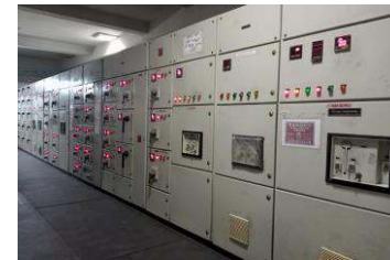
Fig4: LT Breaker Main Incomer at NSAIL
