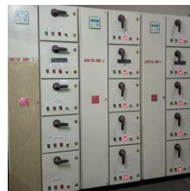
Fig2: Capacitor Bank at NSAIL
