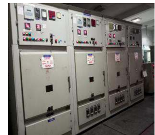
Fig3: HT Breaker Main Incomer at NSAIL
